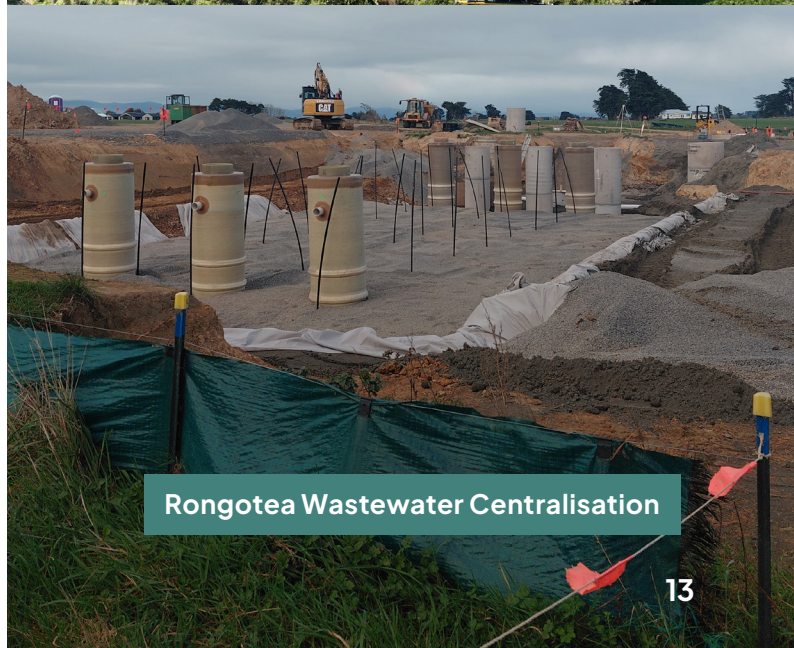
Rongotea Wastewater Centralisation
